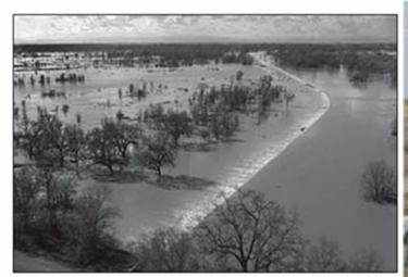
Water from the Sacramento River and Sutter Bypass flow over the Fremont Weir (distinguished by the churning white water) as it heads toward Sacramento, California in February 2004. The Fremont Weir was built in 1924 and was designed to relieve pressure from the Sacramento River when water reaches a predetermined height. Photo by Randy Pench/The Sacramento Bee.
